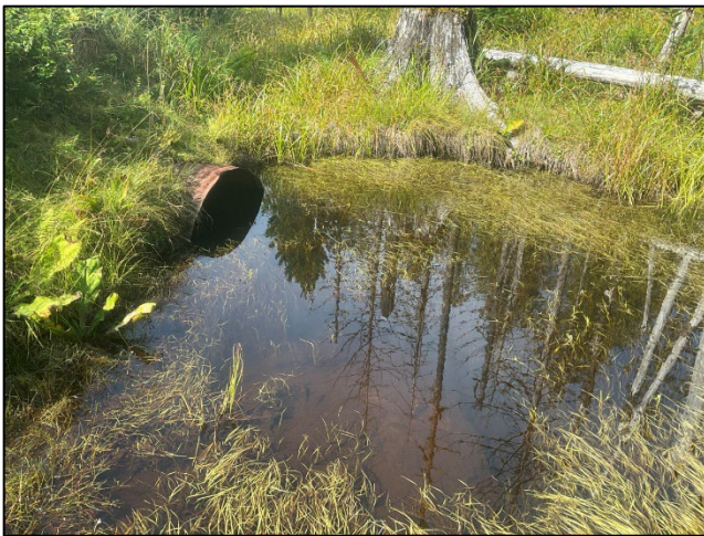
Figure 2.—Backwatered inlet of culvert at waypoint 1001.
